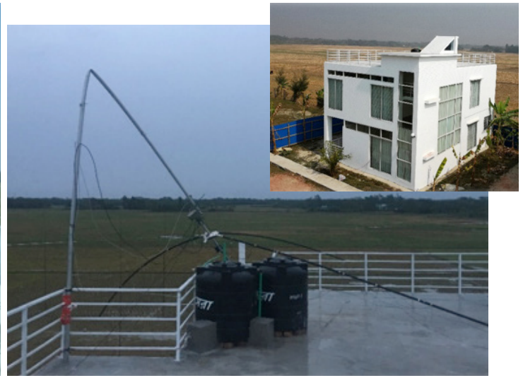
Installing a Spiderbeam antenna on the rooftop (left) of our QTH (upper right), but intense winds ripped out the binding wires, bending the pole.
