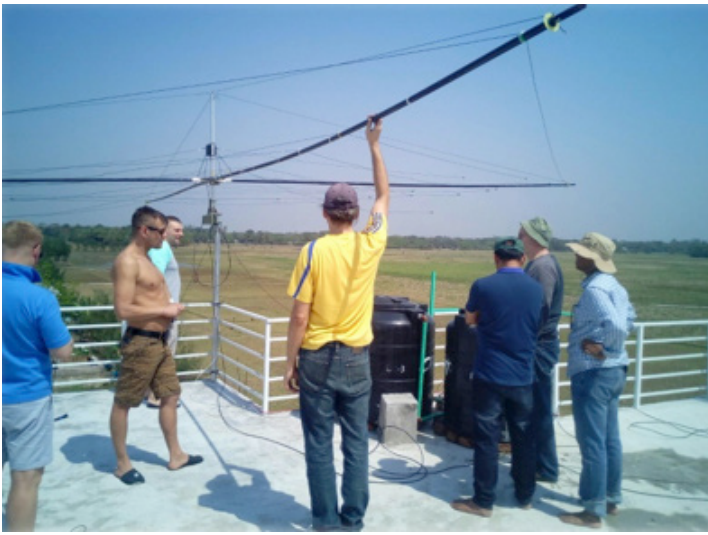
Installing a Spiderbeam antenna on the rooftop (left) of our QTH (upper right), but intense winds ripped out the binding wires, bending the pole.
