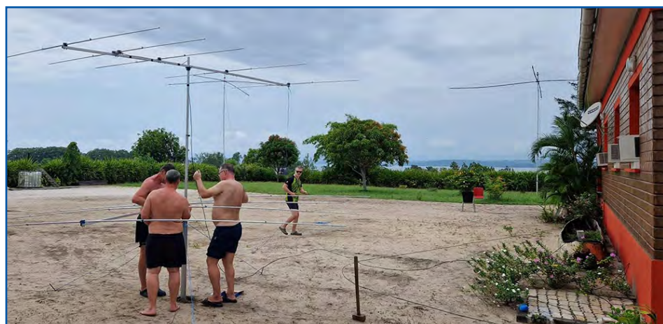
Constructing the antennas.
