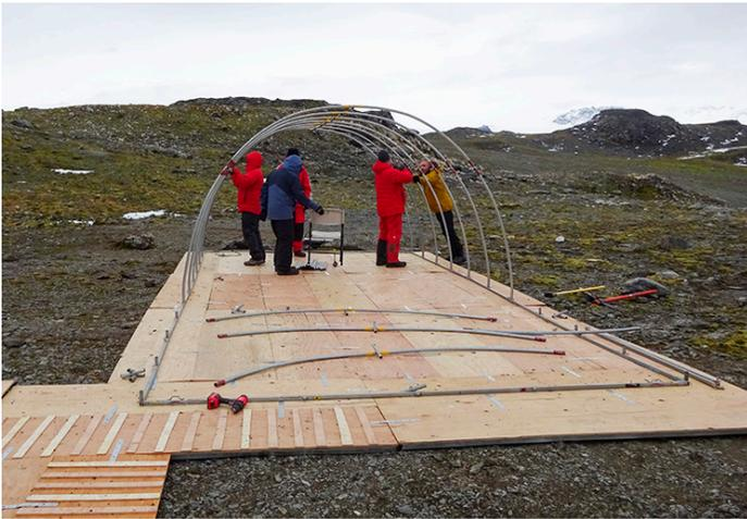
*Prefabricated floor for the Quonset huts. Photo: NG2H*
